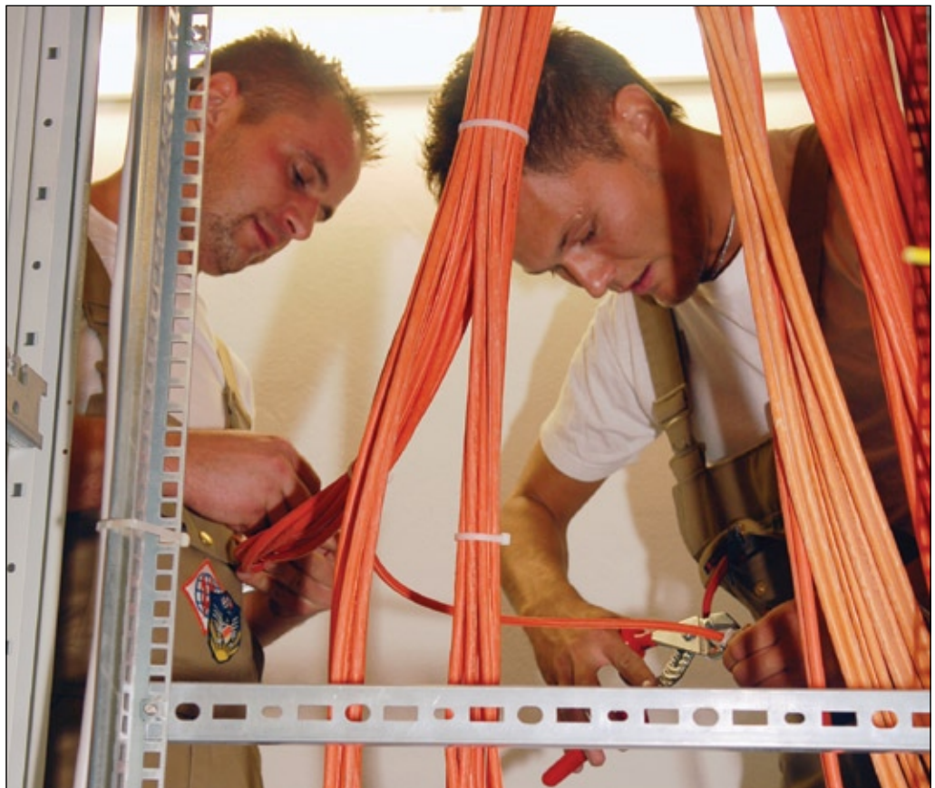
Markus Wuerges, (left), and Matthias Menge (right), both from 2nd Signal Brigade's 6981st Civilian Support Group, splice connectors onto cable that will be used for phone and internet in the new Warrior Transition Unit near the Landstuhl Regional Medical Center.
