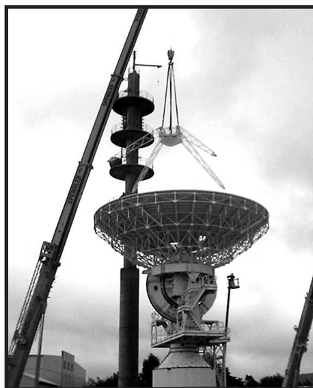
Final installation of the AN/FSC-78B.
