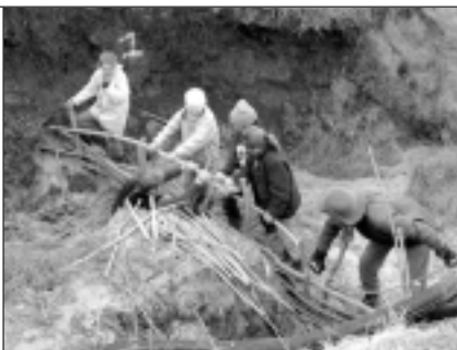
The students lend a hand to install a “willow wall” bank stabilization structure.
