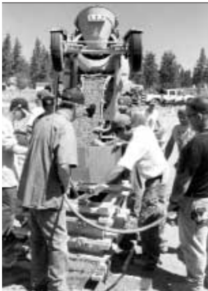
The footings are laid for Turbull’s Environmental Education Center.
