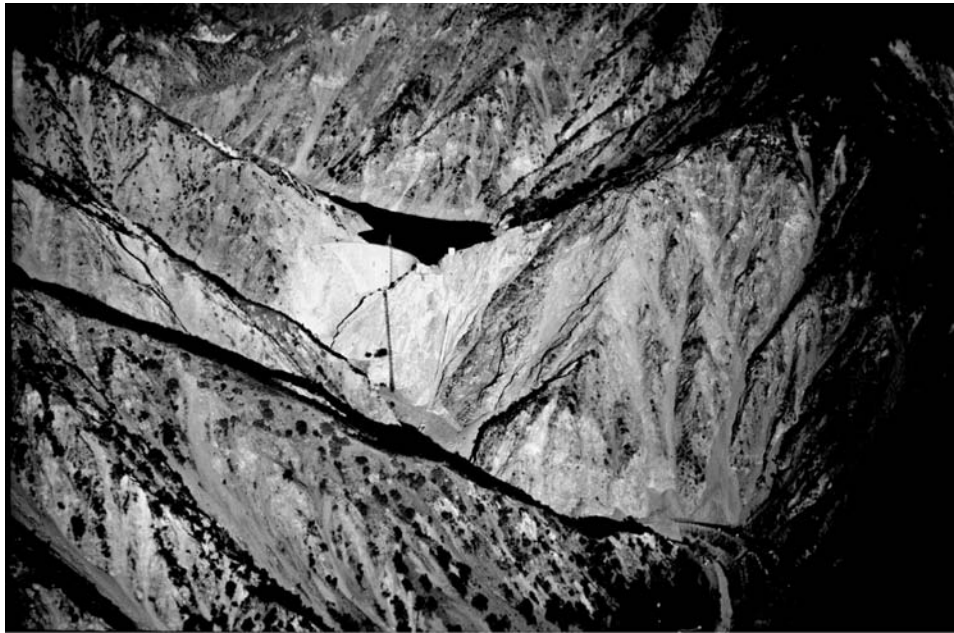
Figure 4. Oblique aerial photograph of Pacoima Canyon and Dam following the 1994 Northridge earthquake showing abundant triggered rock falls on steep slopes.
