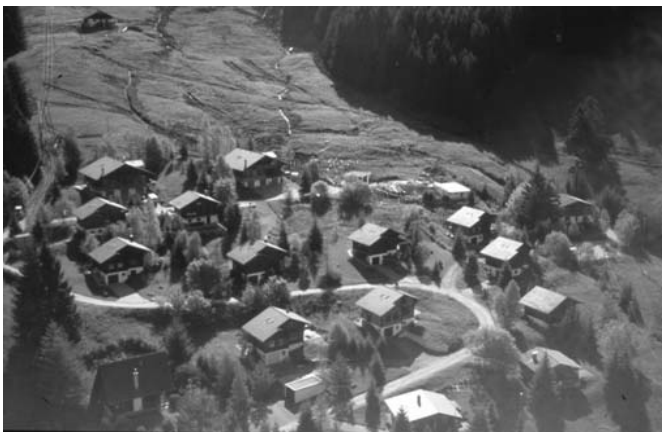
Figure 12. View of the village of Falli Hölli at the beginning of the crisis. These houses moved over more than 200m. Some drainage ditches are seen in the back of the village.
