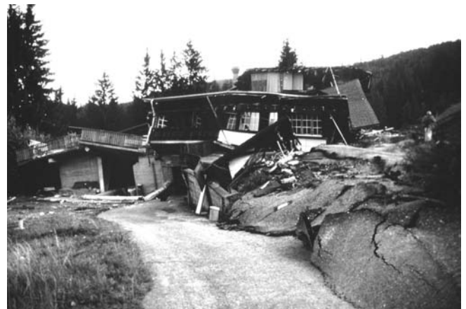
Figure 13. The restaurant was destroyed at the end of July, 1994, due to a shear movement.
