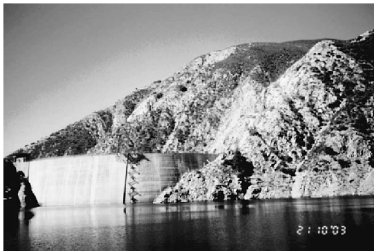
Fig. 2. Pacoima dam and reservoir, and rock mass of the right dam abutment.
