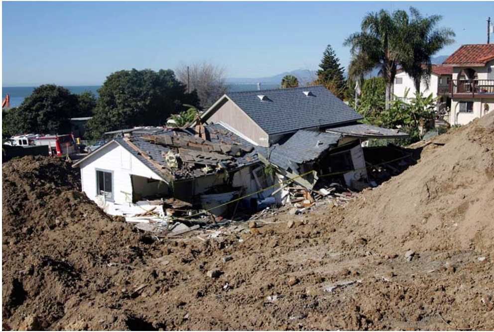
Fig. 9 The 2005 landslide moved as a rapid debris flow, but it was quite viscous and pushed houses in its path rather than flowing around or through them. Debris on the roof of the house is from an adjacent house that was pushed downslope by the landslide
