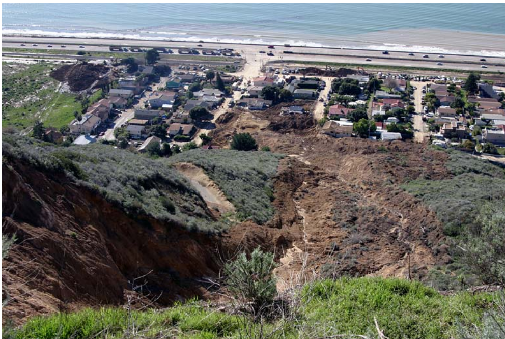
Fig. 6 View from the main scarp down the length of the 2005 La Conchita landslide. Water visible in the center of the photo was issuing from the base of the main scarp when the photo was taken (14 January 2005). The 2005 landslide remobilized about 15% of the 1995 deposit
