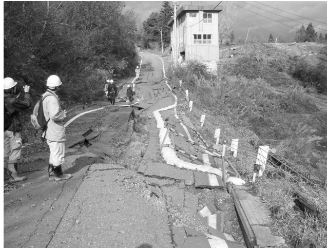
Figure 3. Headscarp of a rotational failure along Highway 23 in the Yamakoshi epicentral area.
