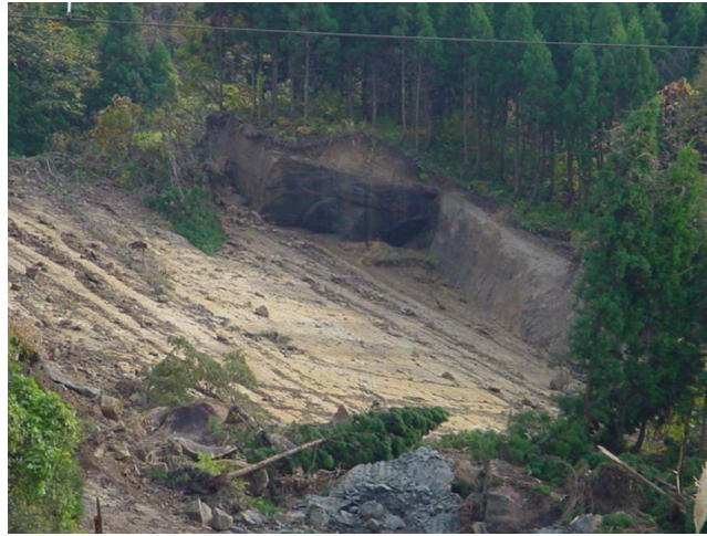
Figure 13. Uragara rock-block slide formed by a bedding plane (sliding surface) and two sets of vertical joint release surfaces.
