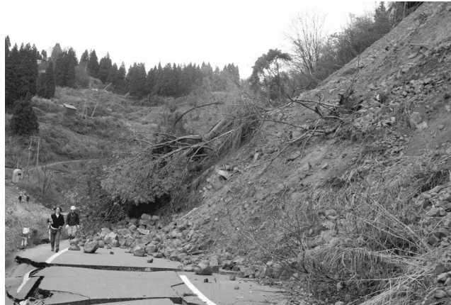
Figure 25. Landslide from a slope above a road east of Yamakoshi.
