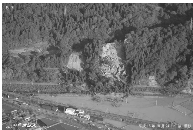
Figure 12. Two adjacent rock-block slides south of Uragara, along Highway 291 (photo: Original Research Ideal Survey, http://www.oris.co.jp/jishin2004/h16jisin_k.htm ).
