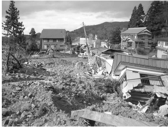
Figure 19. Debris deposited by a northwest-flowing slump-flow complex, with destroyed buildings along the right margin, on Highway 24 northeast of Yamakoshi City Hall.
