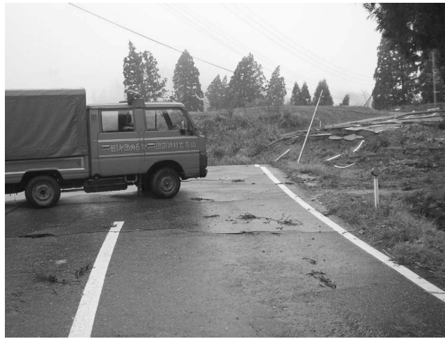
Figure 6. Looking northwest, toward a fire truck that was parked across Highway 291 southeast of Yamakoshi City Hall to prevent vehicles from driving off a headscarp.
