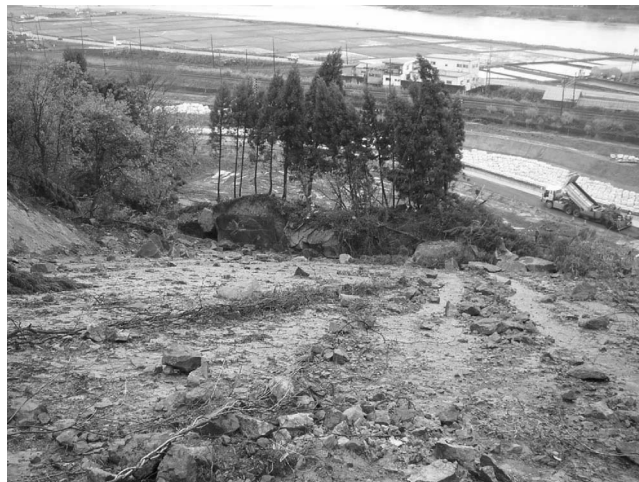
Figure 14. Downslope view of the Uragara slide plane and debris. The Shinano River is in the background.
