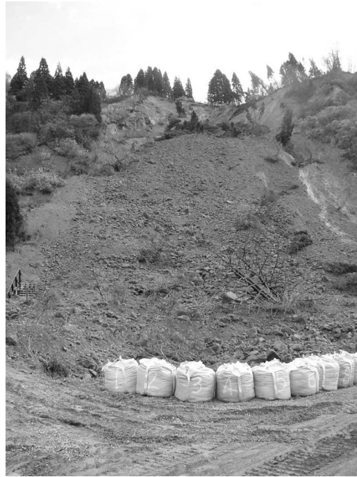
Figure 18. Northwest-facing slump-flow complex with a large headscarp at the top and debris in the foreground, on Highway 24 northeast of Yamakoshi City Hall.
