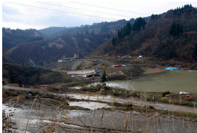
Figure 24. The upstream face of the Komatsugura landslide dam. The reservoir extends upstream to the right. The light gray area in the center left is a spillway being excavated and armored. Note several shallow landslides on the slopes in the background.
