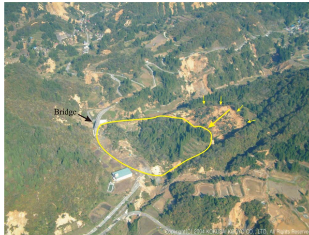
Figure 23. Oblique aerial view of a landslide dam west of Komatsugura before the reservoir filled. The area in the center, which is enclosed by a line, shows the extent of the slide mass; small arrows show the uppermost extent of the main scarp; and the large arrow shows the movement vector. The bridge at left was completely submerged at the time of the reconnaissance, and the reservoir had backed up as far as the village shown in the upper left (photo: Kokusai Kogyo Company, Ltd.).
