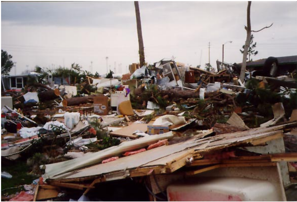
Extensive damage to mobile homes and recreational vehicles at the Ponderosa RV Park in Kissimmee, Florida. Main office building on extreme right of photograph received minor roof damage. Photograph courtesy of Lynn Maximuk.
