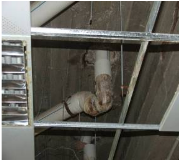
Figure 7 BPA Improper Plumbing Installation in cadets' barracks and expansion crack on rear side of instructors' barracks
