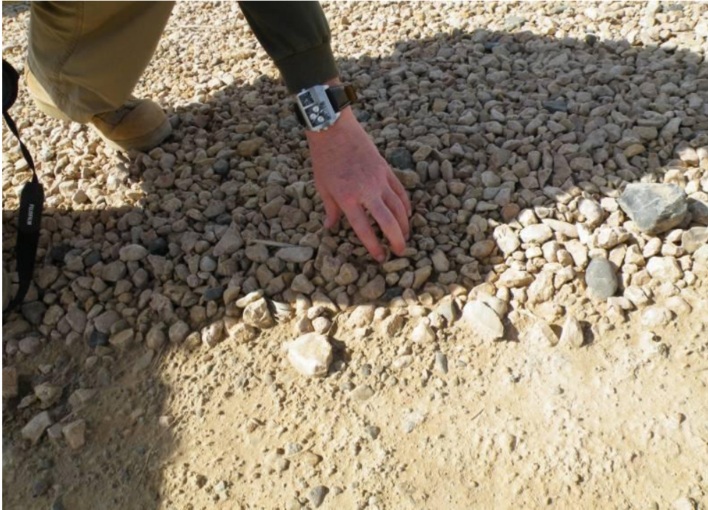
Site Photo 10. Roadway surface
