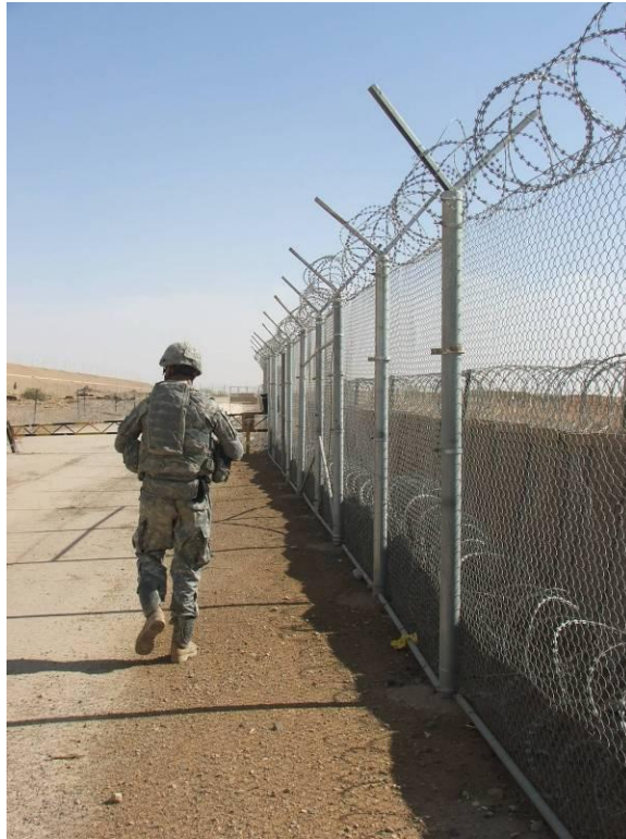
Site Photo 2. Typical fence section
