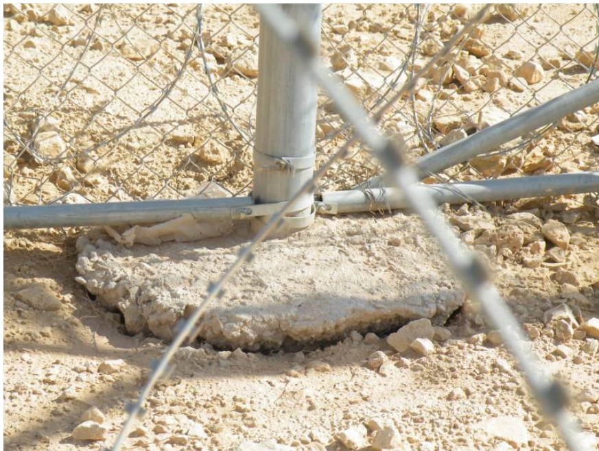
Site Photo 7. Concrete anchorage
