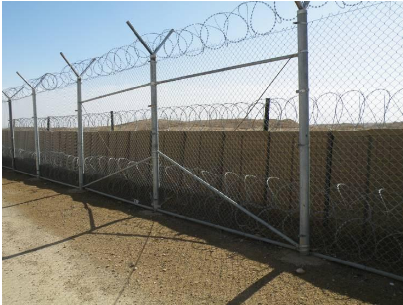
Site Photo 3. Typical fence section
