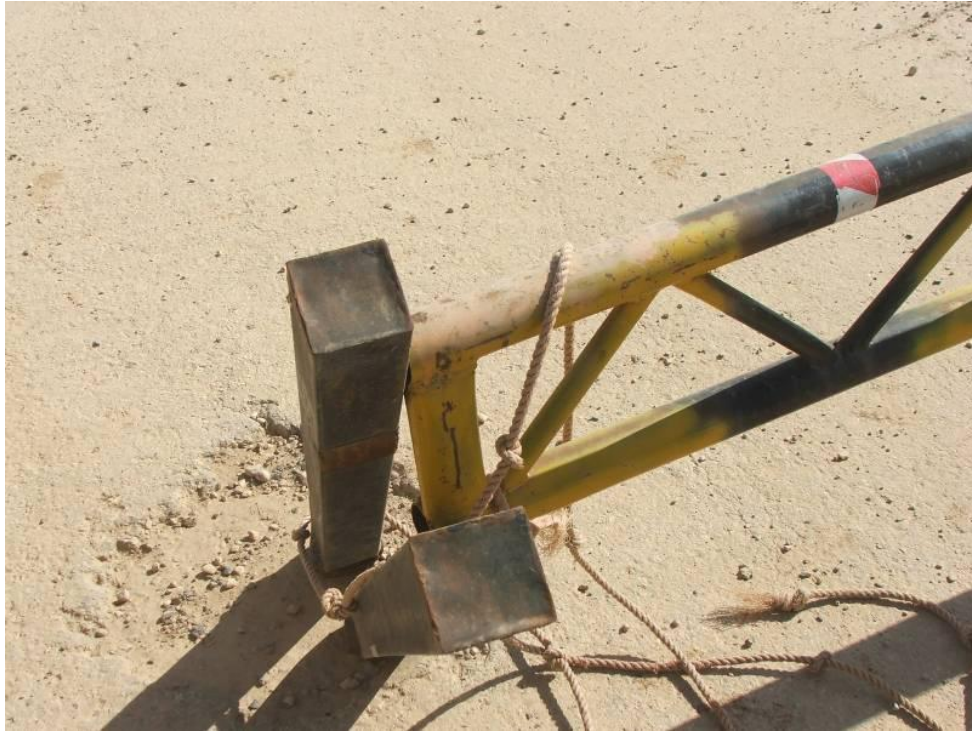
Site Photo 13. Misaligned lifting gate
