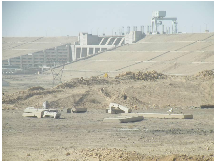
Site Photo 1. Haditha Dam
