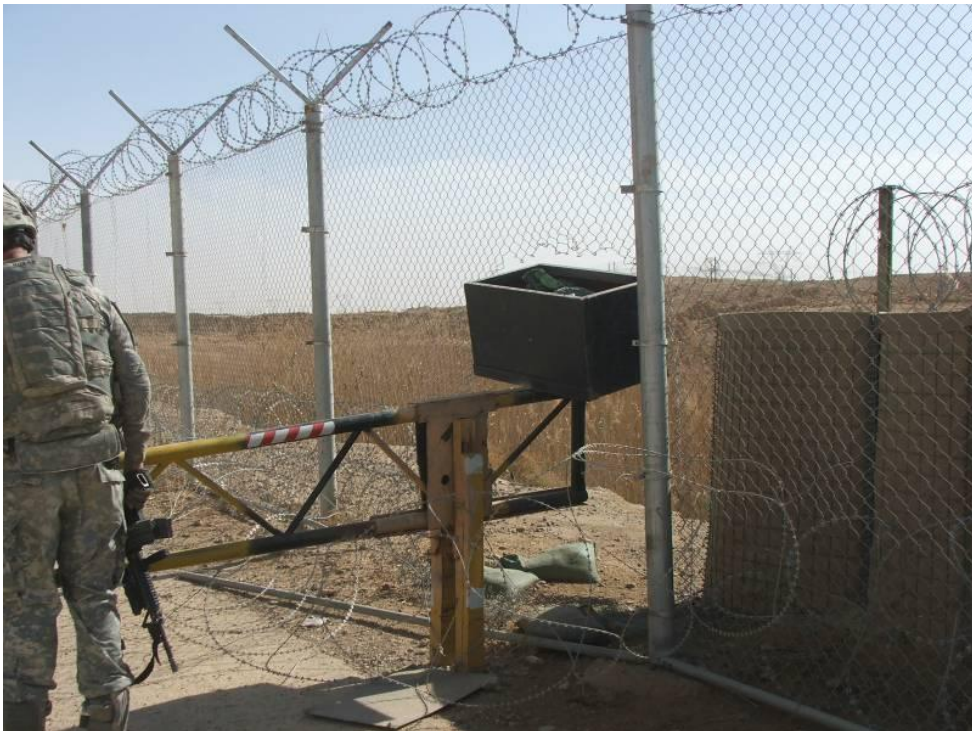
Site Photo 14. Lifting gate with modified fence
