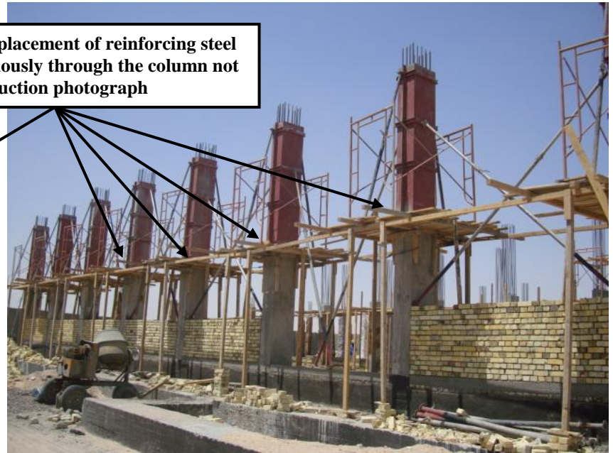
Site Photo 6. Form construction for columns without placement of intermediate tie beams (Courtesy of GRS)
