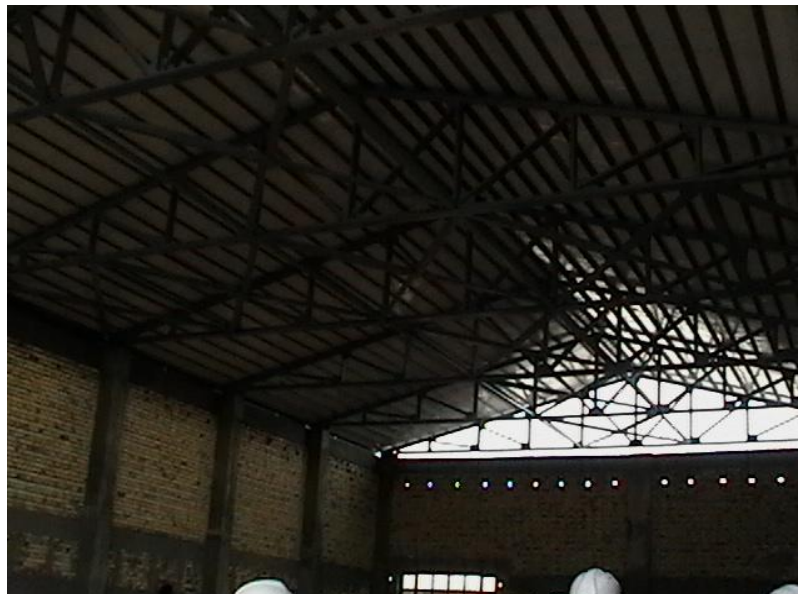
Site Photo 7. Slaughtering building with top beam and column connections (Courtesy of GRS)
