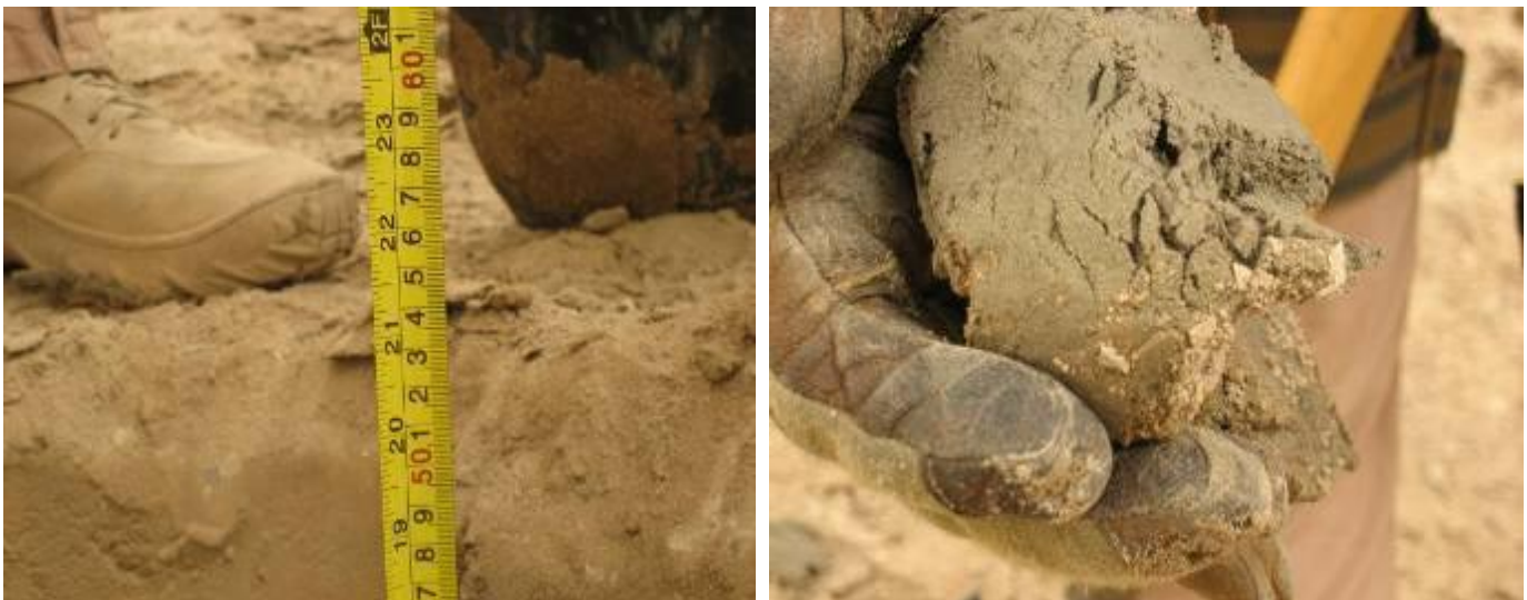
Site Photos 1 and 2. Site survey found clay at a depth of less than two feet (Courtesy of GRS)
