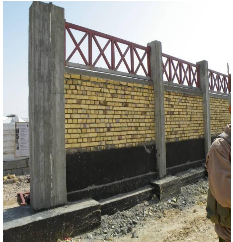
Site Photo 3. Partially constructed perimeter fence
