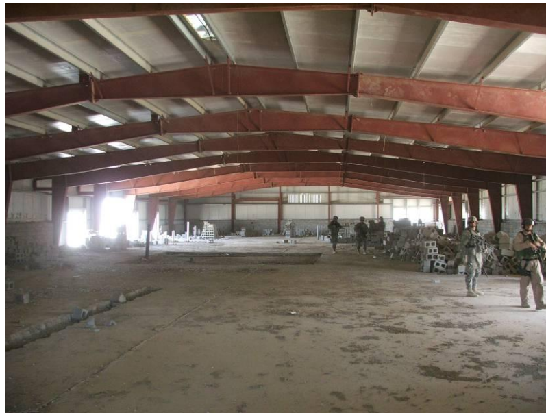
Site Photo 26. Interior of partially completed prefabricated building
