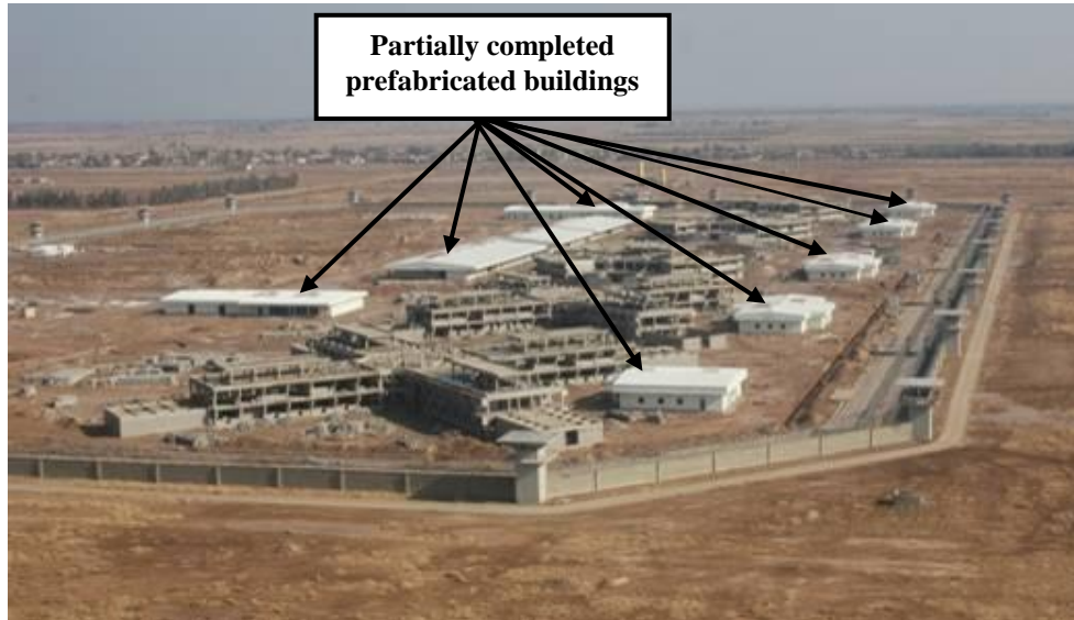
Site Photo 25. Aerial view of KBS Correctional Facility (Courtesy of the USAACE)
