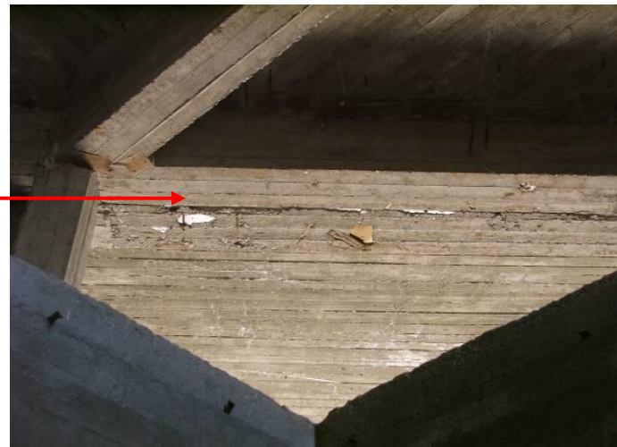
Site Photo 11. Roof from medium security building
