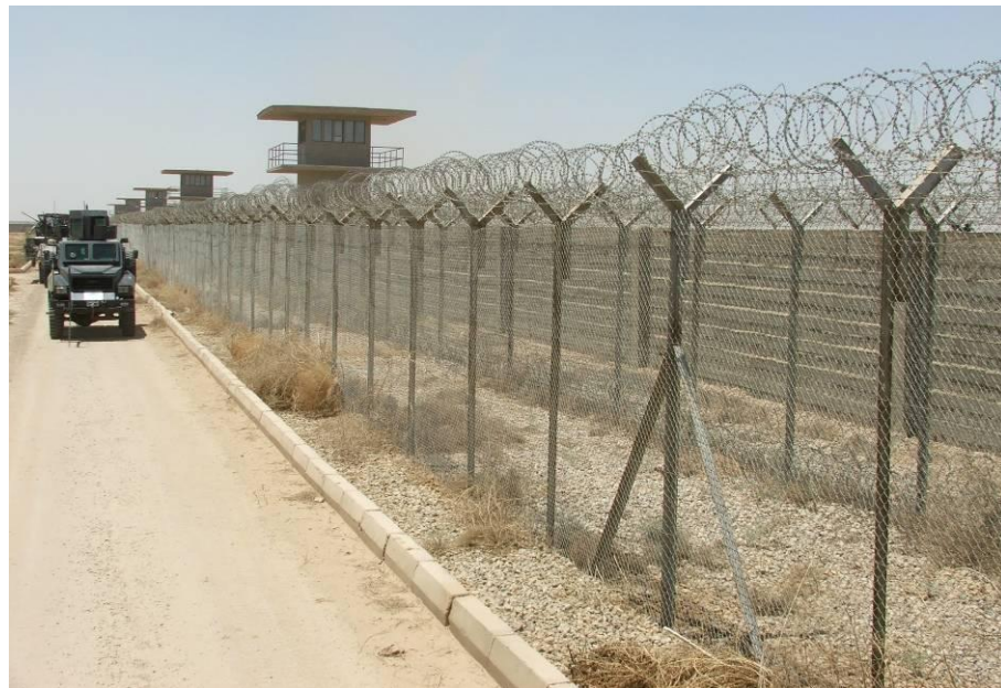
Site Photo 24. Interior fence
