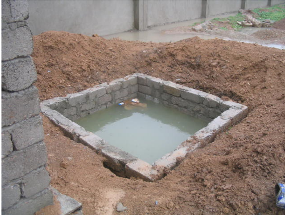
Site Photo 9. Septic tank testing (Photo courtesy of USACE)
