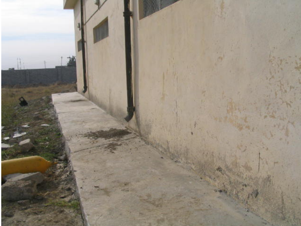
Site Photo 5. New recast walkway (Photo courtesy of USACE)
