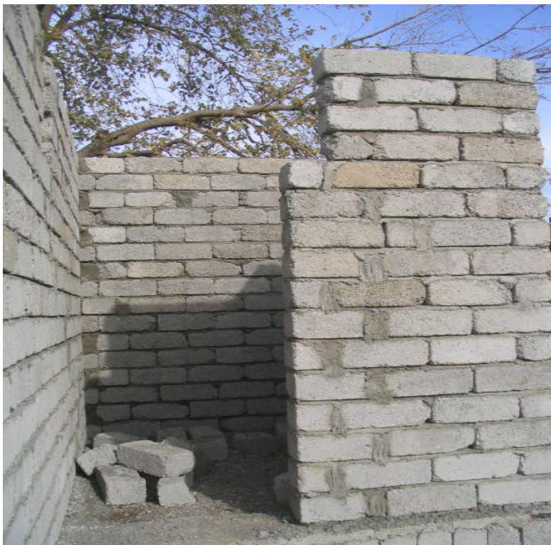
Site Photo 6. Construction of a water closet (Photo courtesy of USACE)
