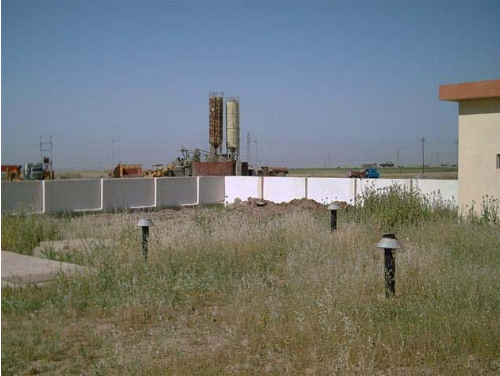
Site Photo 13. Newly constructed security wall (Photo courtesy of USACE)
