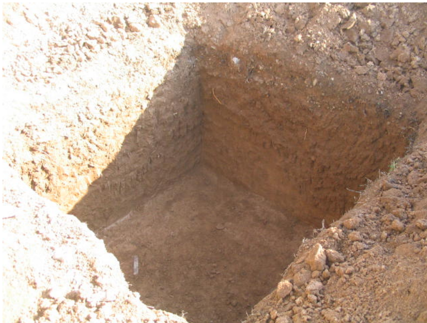
Site Photo 8. Excavation of septic tank (Photo courtesy of USACE)
