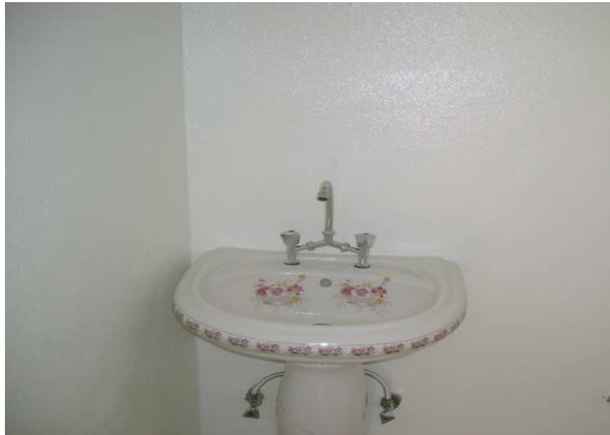
Site Photo 7. Completed construction of water closet (Photo courtesy of USACE)
