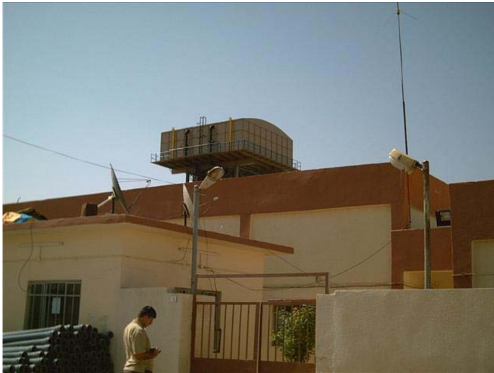
Site Photo 4. General maintenance performed on the exterior of the Bartilla Booster Pump Station (Photo courtesy of USACE)
