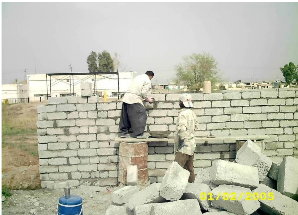
Site Photo 12. Construction of security wall (Photo courtesy of USACE)
