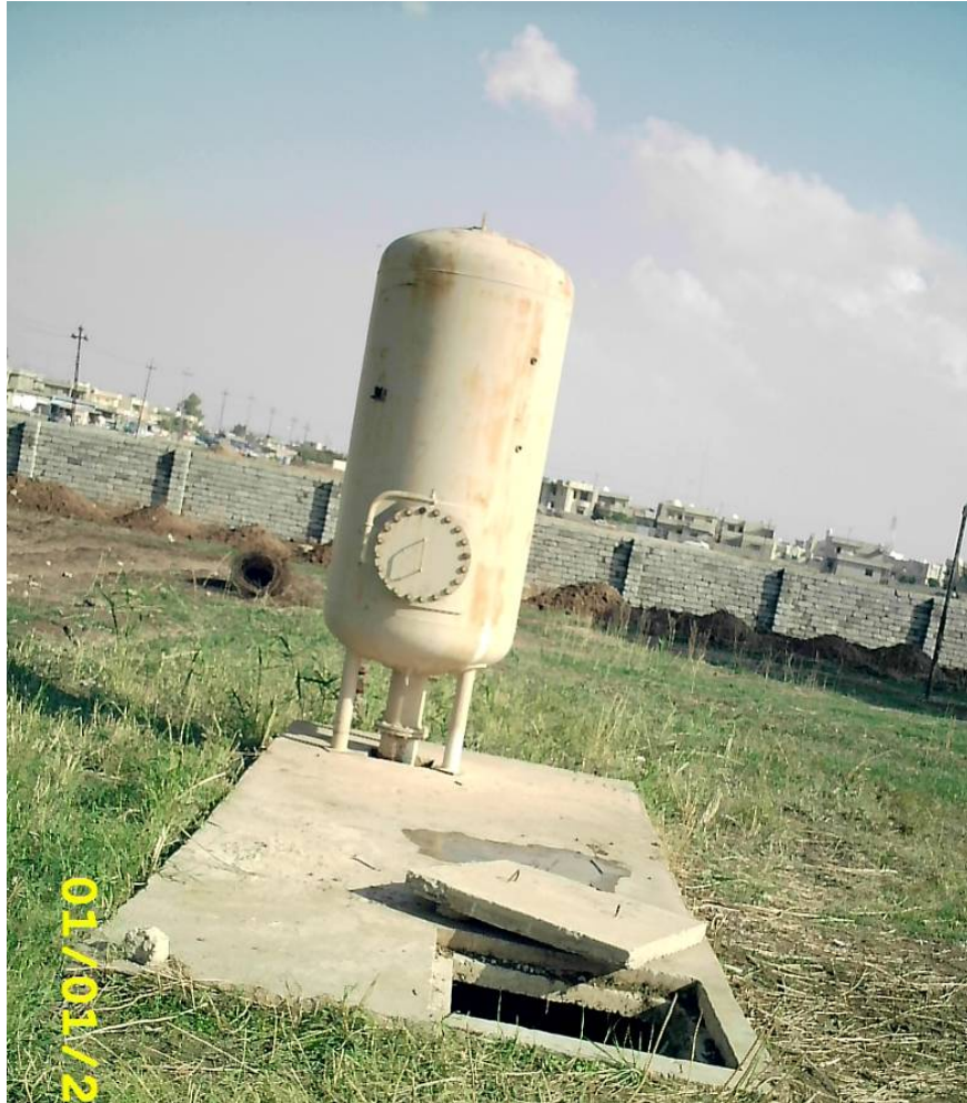
Site Photo 1. Anti-Hummer system before maintenance (Photo courtesy of USACE)
