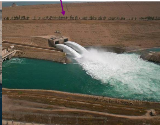
Site Photo 3. Close up of bottom outlet (Photo courtesy of the USACE)
