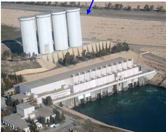
Site Photo 2. Close up of hydroelectric power plant (Photo courtesy of the USACE)
