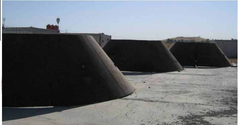
Site Photo 22. Three partially welded funnels for the stationary silos
