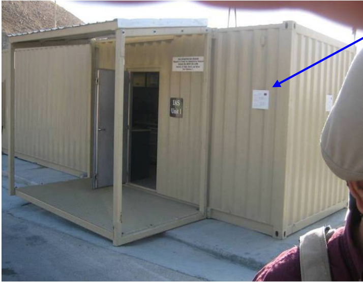
Site Photo 27. Exterior view of an IAS unit
