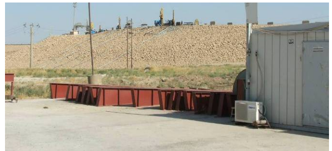
Site Photo 23. Miscellaneous pieces of metal for the stationary silos
