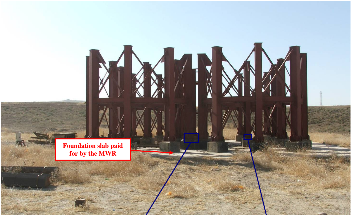
Site Photo 17. View of the partially constructed stationary silos
