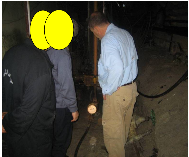
Site Photo 45. A hole being actively grouted (Photo courtesy of ITAO)
