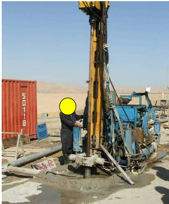
Site Photo 41. Dam personnel conducting above ground drilling operations
