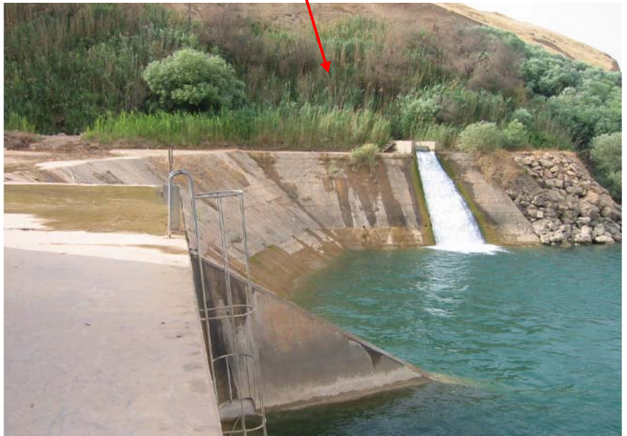
Site Photo 7. Close-up view of seepage at the Mosul Dam (Photo courtesy of USACE)
