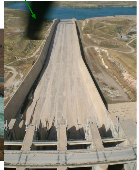
Site Photo 4. Close up of spillway (Photo courtesy of the USACE)
