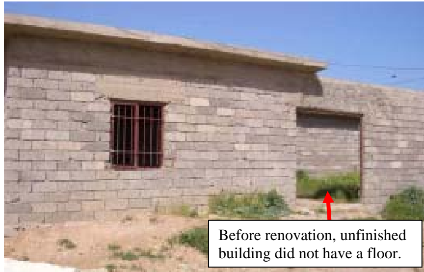
USACE Pre-Construction Photo 2.
