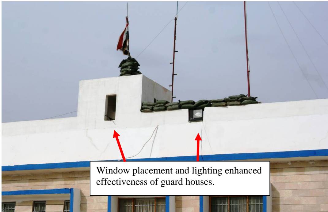
Site Photo 5. As required, new rooftop guard houses and lighting upgrades improved force protection capability.
