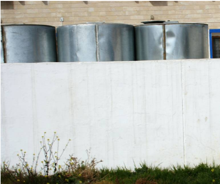
Site Photo 4. Throughout the facility, SIGIR observed new water storage tanks to meet SOW requirements to provide adequate supply.
