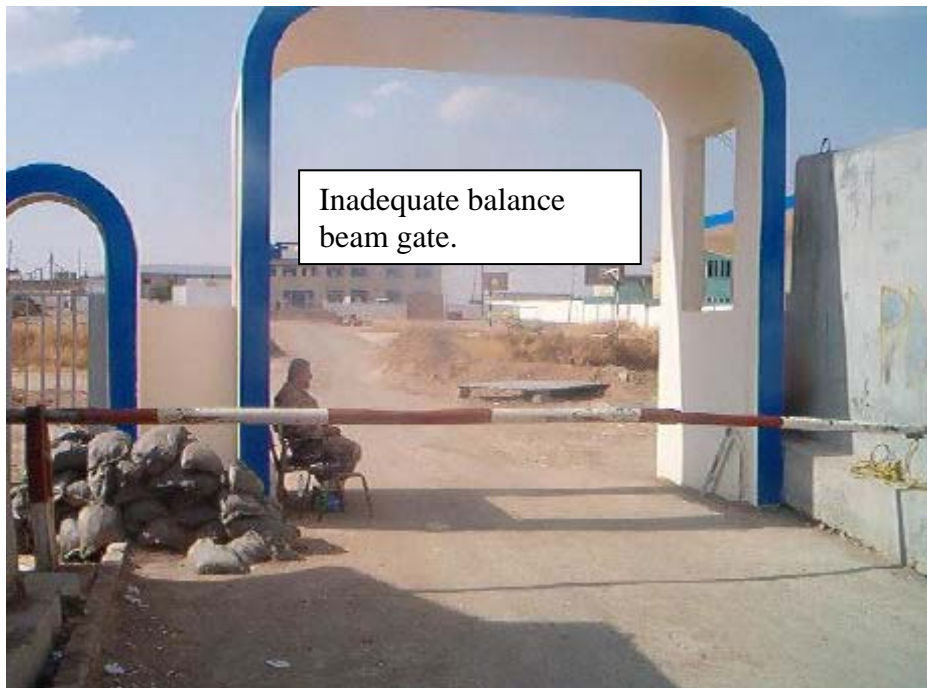
USACE Pre-Construction Photo 3.
