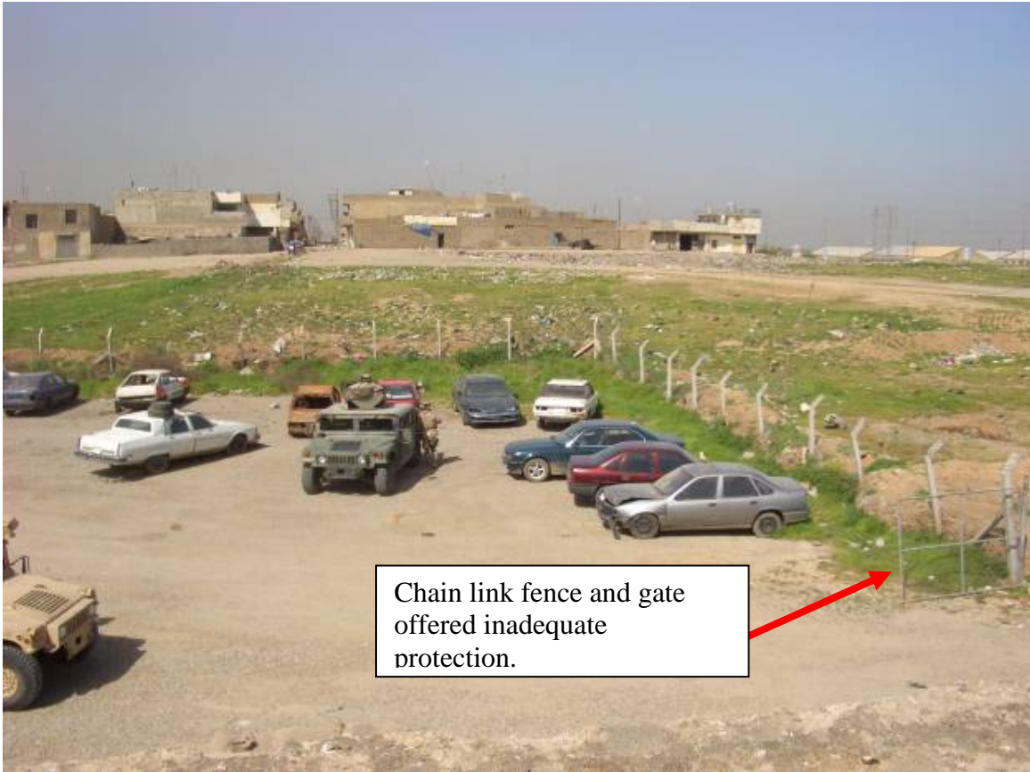
USACE Pre-Construction Photo 3. Without a solid block wall, police station was vulnerable to direct fire and tactical observation from nearby buildings and open fields.
