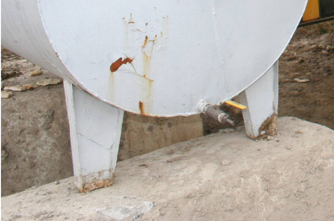
Site Photo 10. Fuel line between the tank and the generator engine had been removed.
