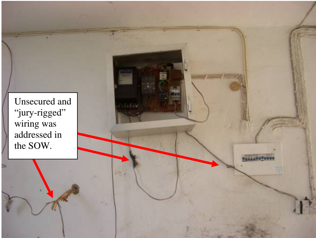
USACE Pre-Construction Photo 6.
