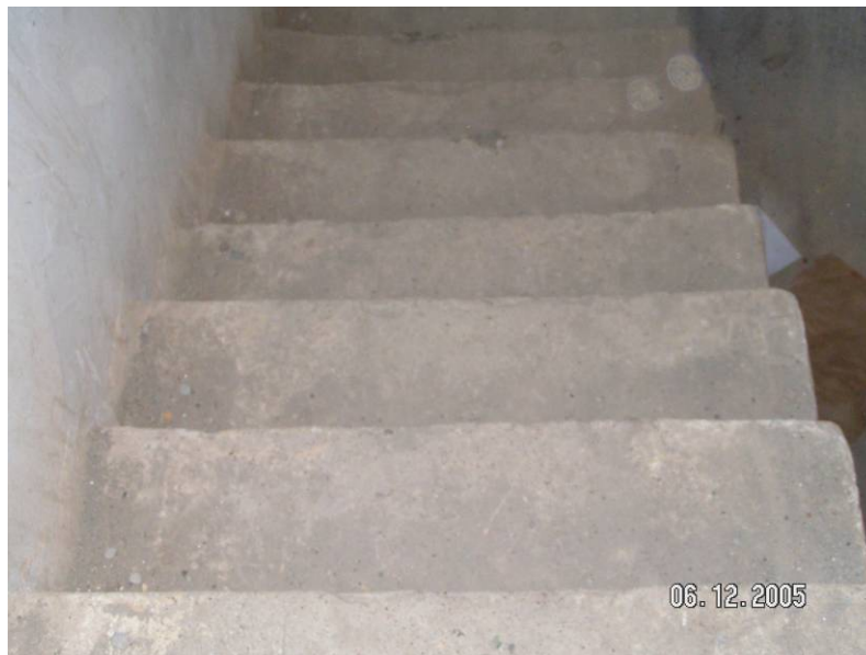
USACE Pre-Construction Photo 8. Before renovation, steps were bare, unsealed concrete.
