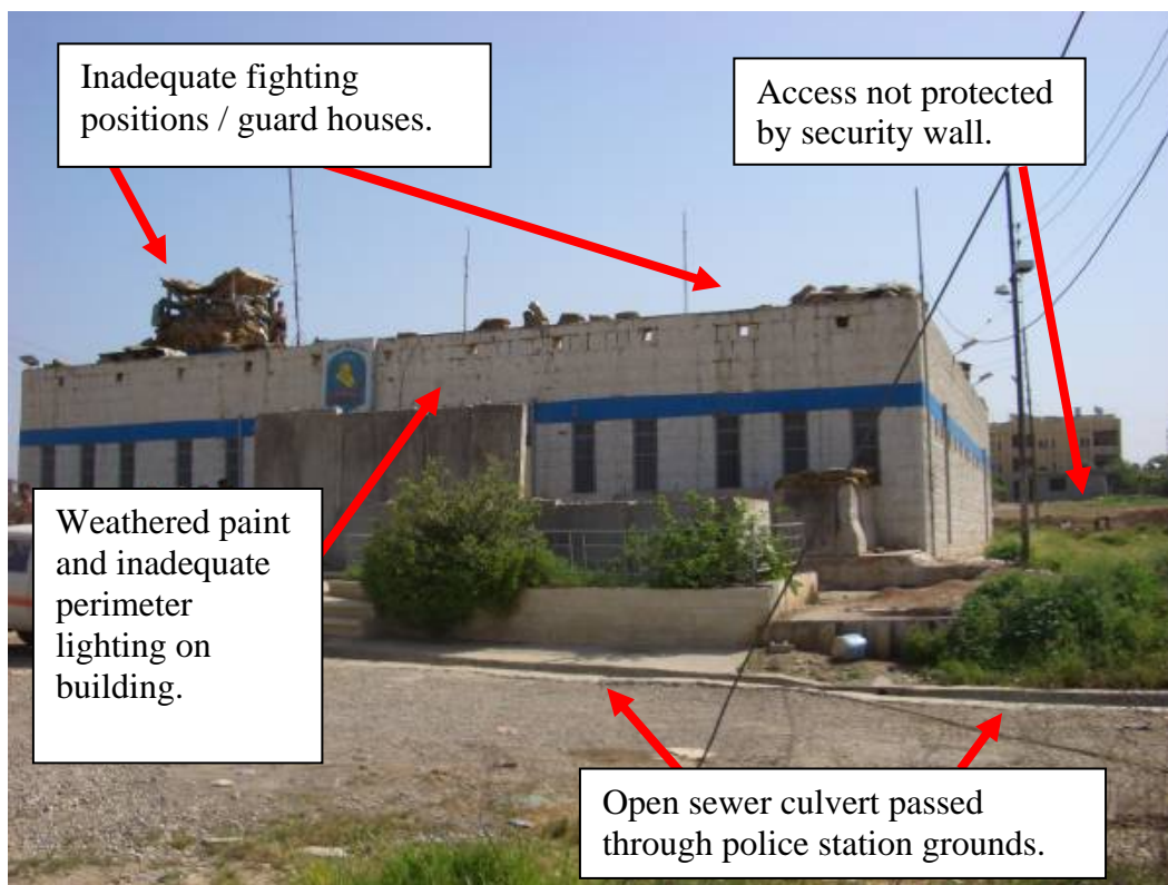
USACE Pre-Construction Photo 1.
