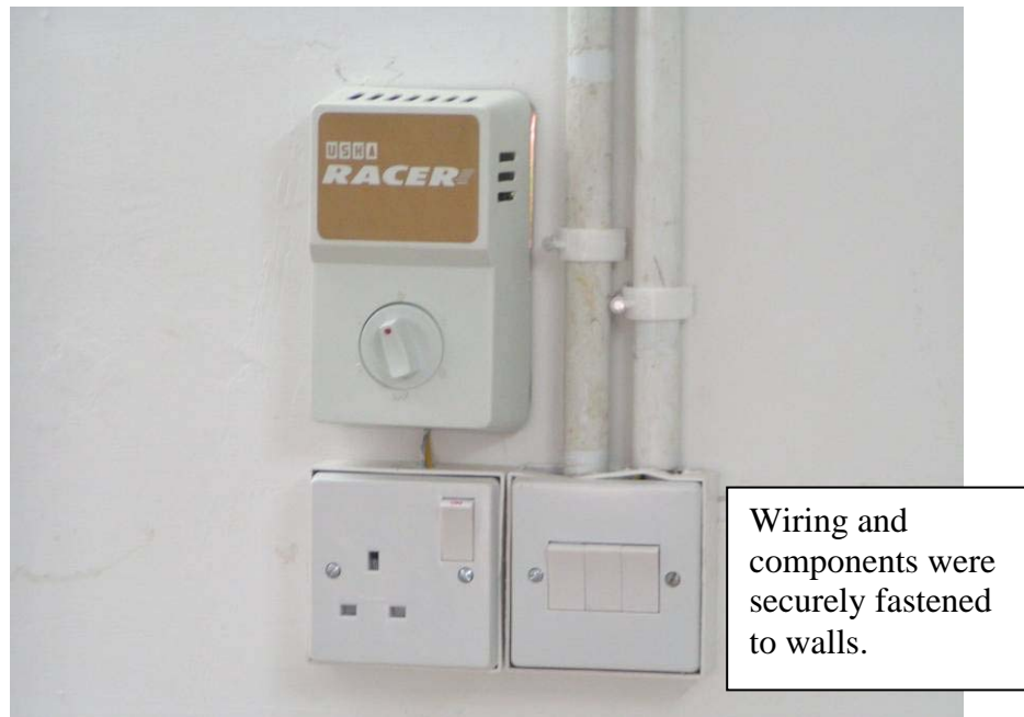
USACE Construction Photo 8 (12 Jun 05)
