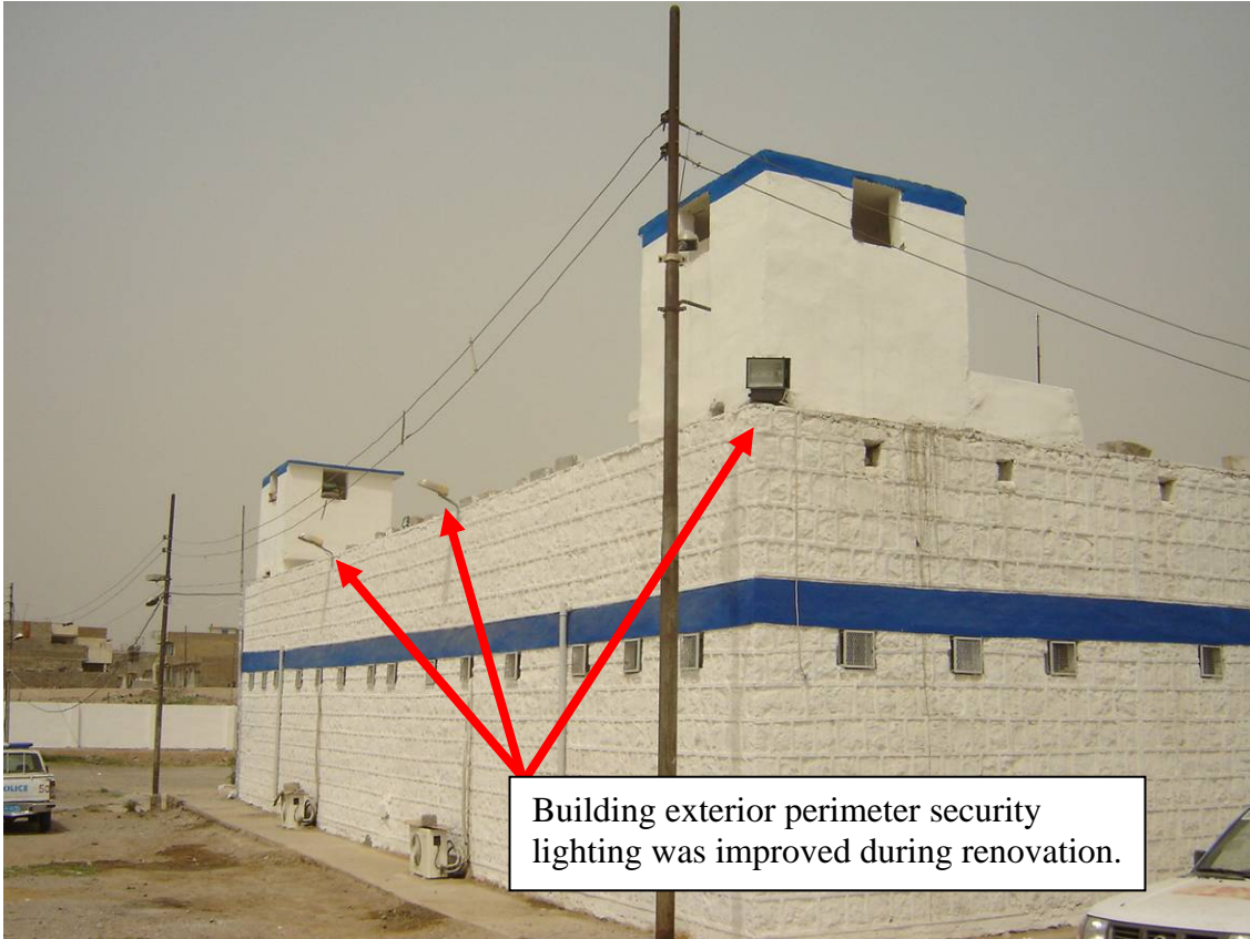
USACE Construction Photo 9 (11 Aug 05)
