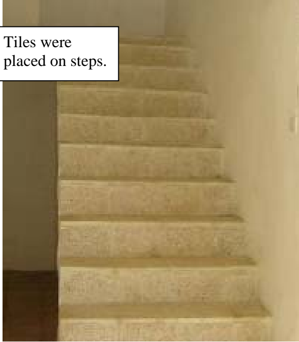
USACE Construction Photo 12 (15 Aug 05)
