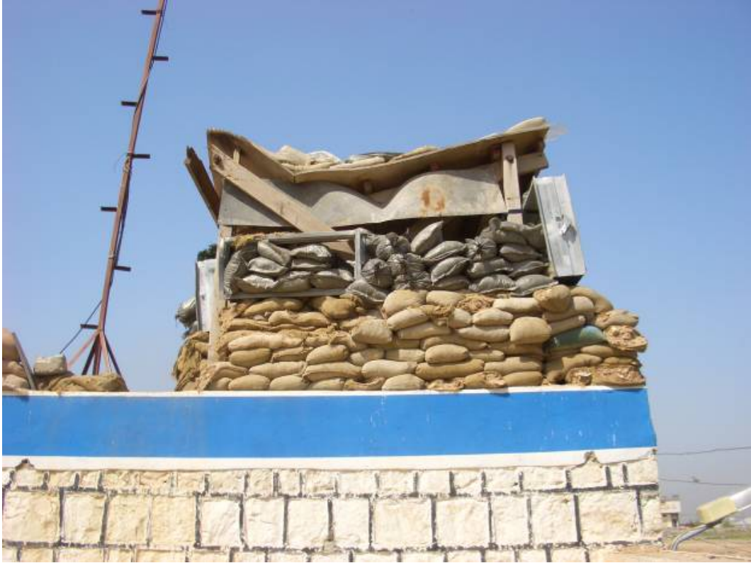
USACE Pre-Construction Photo 5. Rooftop fighting positions/guard houses before renovation.
