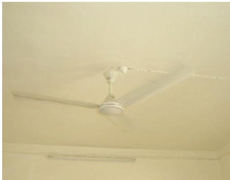
USACE Construction Photo 11 (15 Aug 05)
