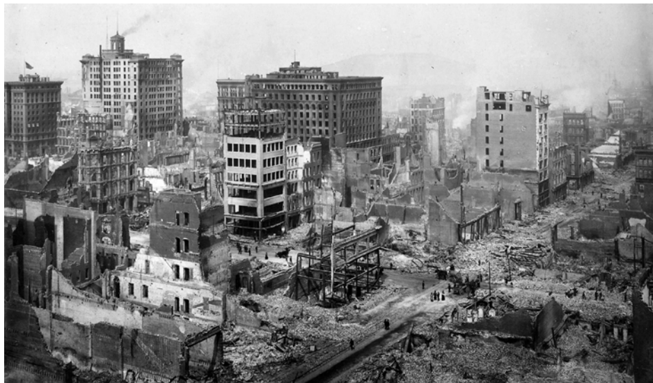
Figure 2-5 - Steel frame buildings in downtown San Francisco performed well in the 1906 earthquake.
