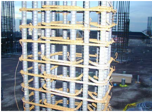
Figure 7-4 – Column cage with hoops constructed from single reinforcing bar.
