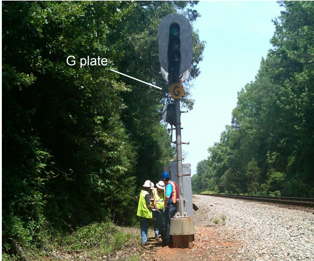
Figure 3. NTSB signal investigators inspecting signal at MP 316 with attached G plate.
