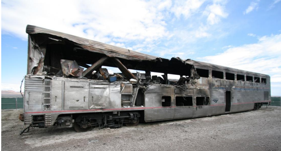
Figure 6. Photograph of first coach railcar 34033 at impound lot, with front of railcar at left, showing extent of damage caused by collision with first side-dump trailer and fire damage throughout railcar.
