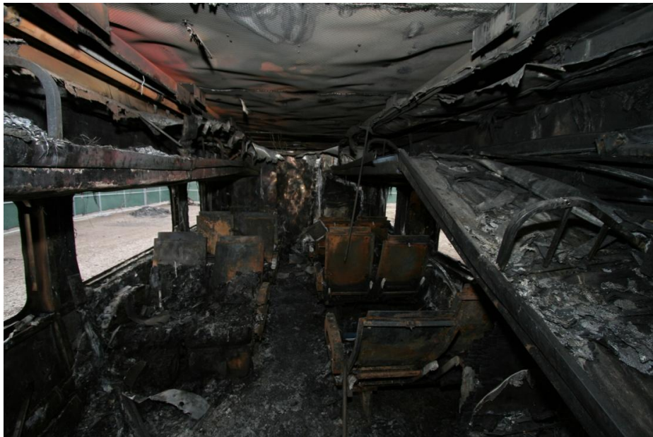
Figure 7. Photograph of interior of lower level of first coach railcar 34033, showing extensive structural and fire damage.
