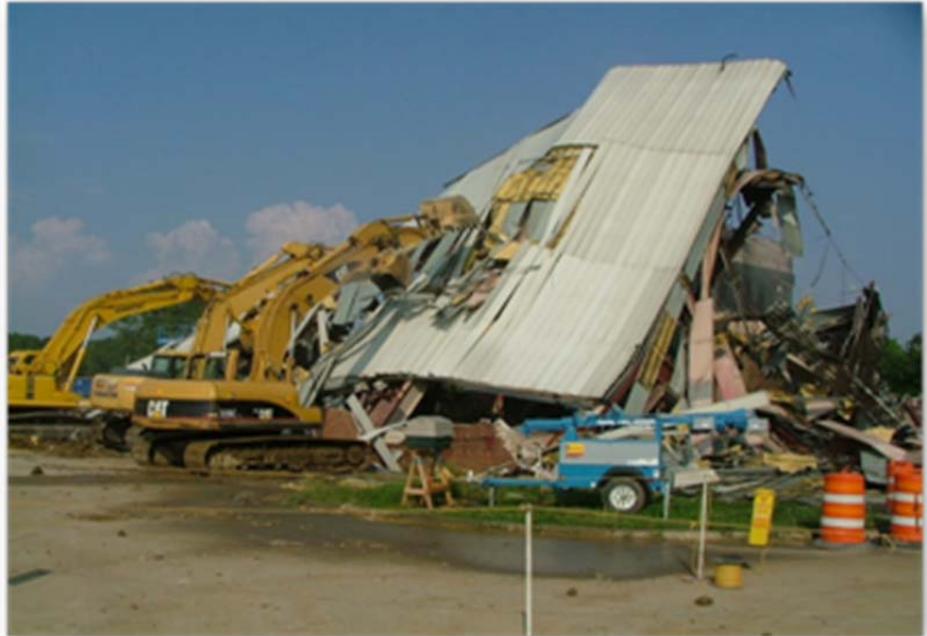
Decontamination & Decommissioning (D&D) at the Columbus Closure Project
