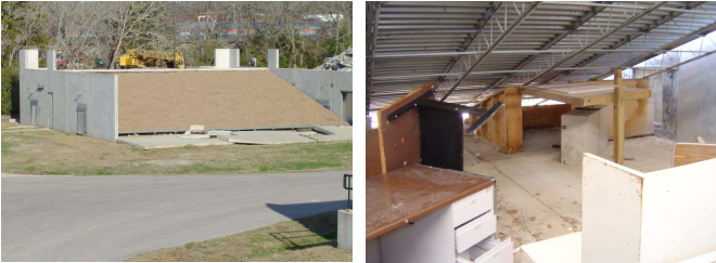
The House of Pancakes collapse scenario
