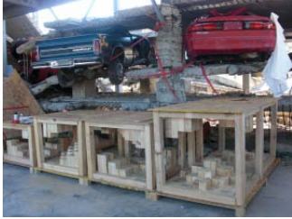
Confined Space Test Method
