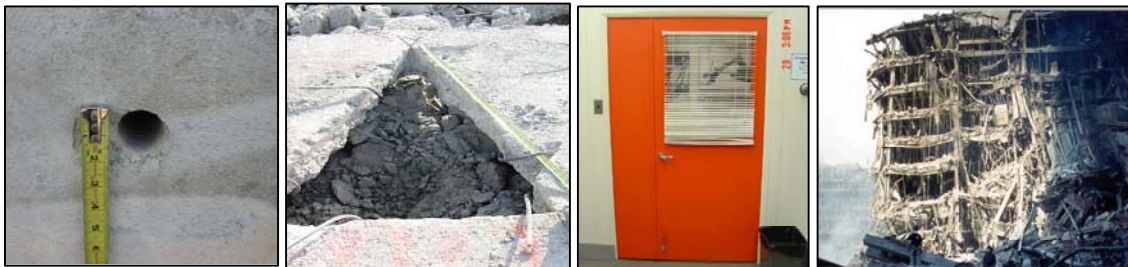
Figure 3: Initial access categories: 2 inch bore hole, 24 inch triangular hole, doorway, and aerial.
