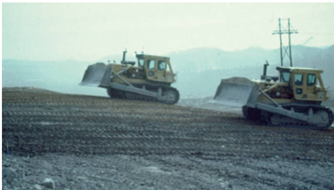
Photo 4. Soil compaction due to equipment operation on mine soils hinders survival and growth of planted trees. "Tracking in" operations, such as those shown in the photo, are NOT recommended for mine sites on which trees will be planted, unless required to stabilize steep slopes.
