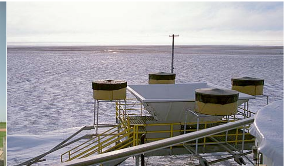
Radar wind profiler
