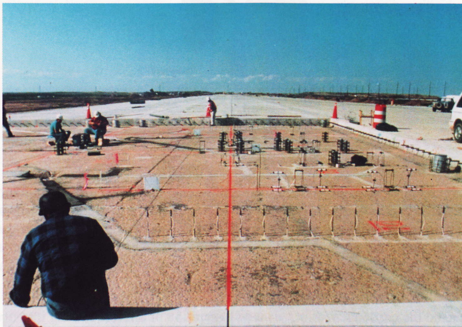
Figure 1. Installation of pavement instrumentation at the new Denver International Airport.
