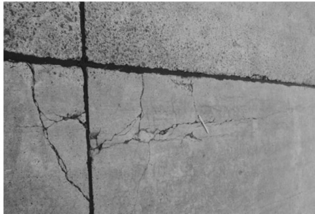
FIGURE 2-28. CORNER SPALLING
