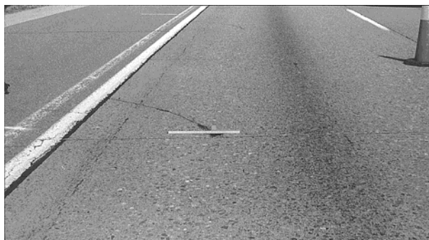
FIGURE 2-14. CORNER BREAK
