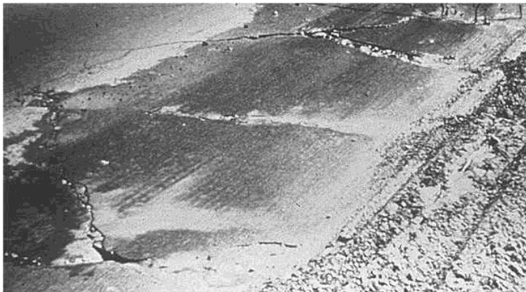
FIGURE 2-22. WATER BLEEDING AND PUMPING
