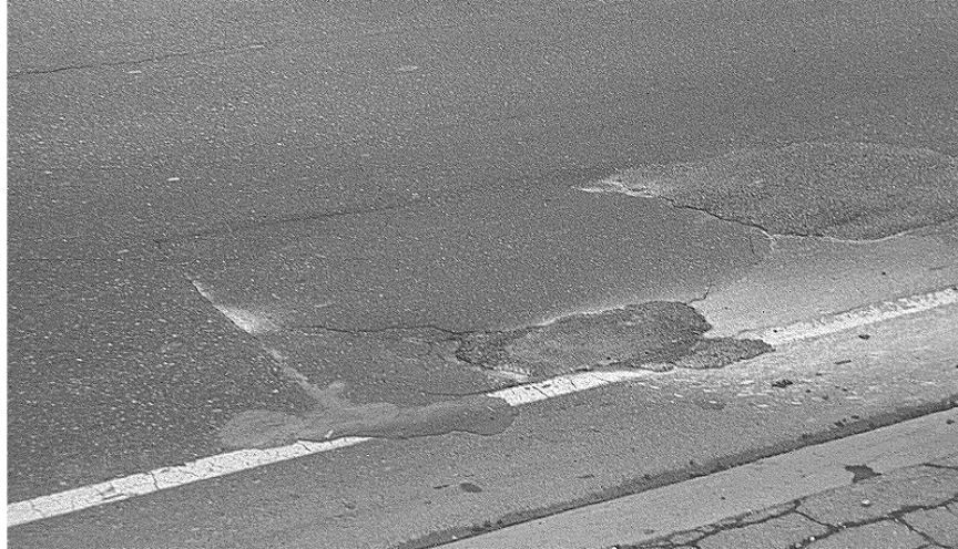
FIGURE 2-7. HIGH-SEVERITY PATCH
