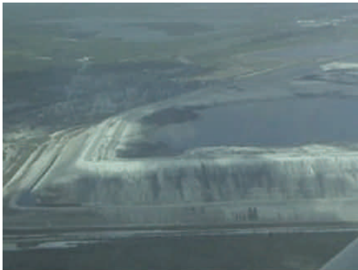
Figure 3. The gypsum walls containing the wastewater are seen in this image taken before the collapse. ( http://www.fluoridealert.org/phosphate/ )
