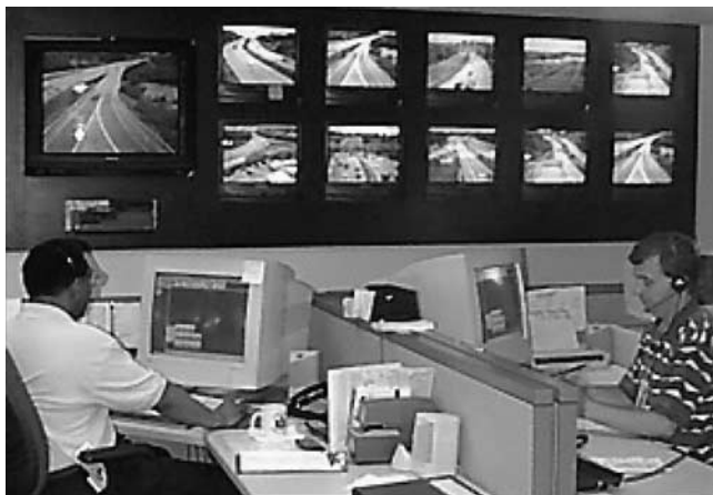
Figure 2. The Transportation Management Center.
