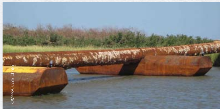
(L) Spraying dredged sediment directly onto broken marsh can deliver nutrients needed for rebuilding. (R) Simple in concept, pipelines carrying sediment to project sites pose engineering challenges: how large its diameter, how wet the slurry, how powerful its pumps, how heavy its weight on fragile marsh soils are but a few of the initial parameters to consider.
