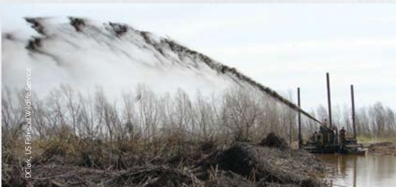
(L) Spraying dredged sediment directly onto broken marsh can deliver nutrients needed for rebuilding. (R) Simple in concept, pipelines carrying sediment to project sites pose engineering challenges: how large its diameter, how wet the slurry, how powerful its pumps, how heavy its weight on fragile marsh soils are but a few of the initial parameters to consider.
