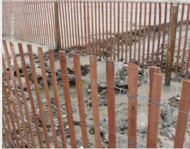
(L) Vegetative plantings and sand fencing are simple measures that work with nature to stabilize the landscape. (C) Even simple measures undergo testing and evaluation to determine how to maximize their effectiveness. (R) Ongoing experiments improve planting techniques and develop superior strains of marsh vegetation.
