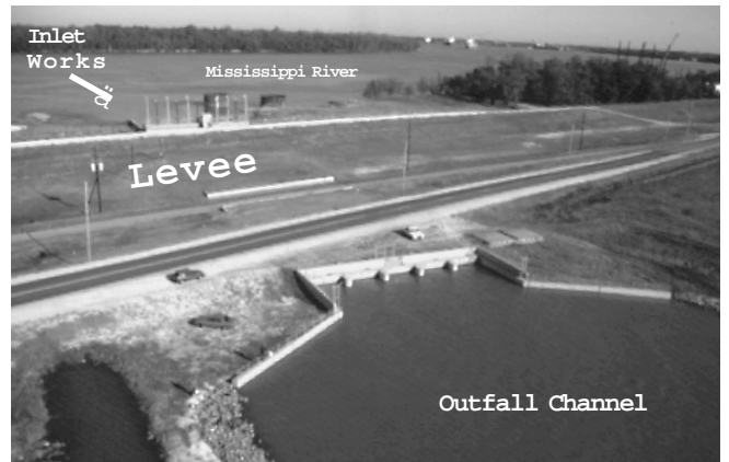
The photo above shows the Caernarvon structure from a reverse angle with the river and New Orleans far in the background.
