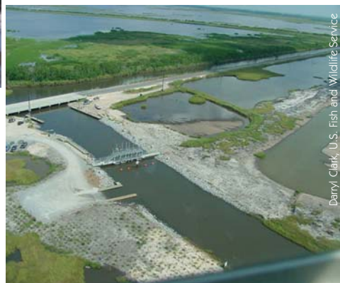
Right: Straddling a small waterway that connects the Sabine National Wildlife Refuge to Calcasieu Lake, the Hog Island Gully water control structure helps protect over 42,000 acres of marsh from high-salinity salt water.
