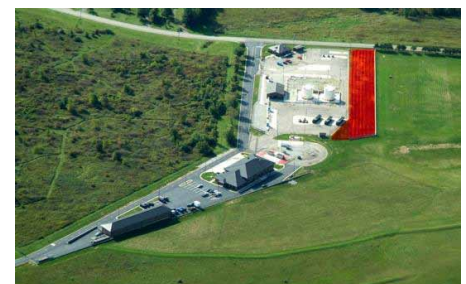
Landfill Gas to Energy Production Facility
