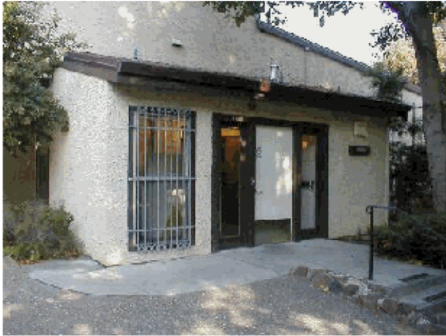
A Sliding Door Was Replaced With A Door That Requires Code Access at Pilgrim Park's Laundry Room
