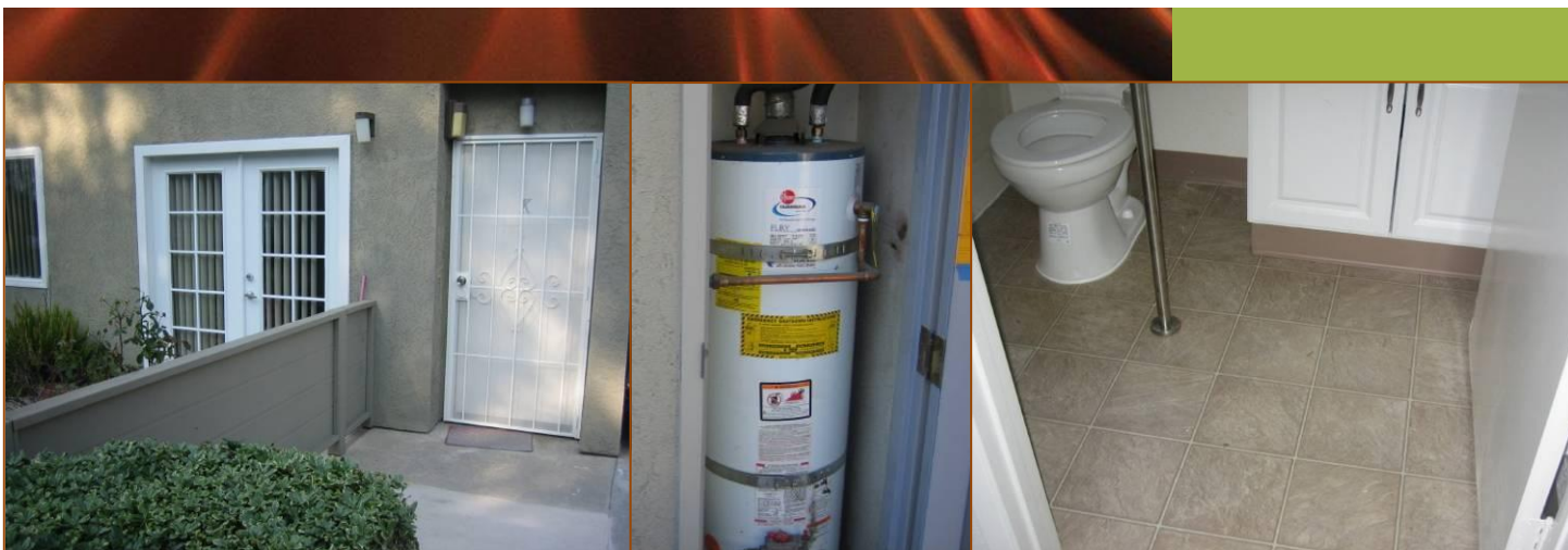
From Left: Outside view of one of 12 new senior housing units completed as part of the McNeill Manor Improvement Project, an example of a new water heater, and vinyl flooring that was used in all units.
