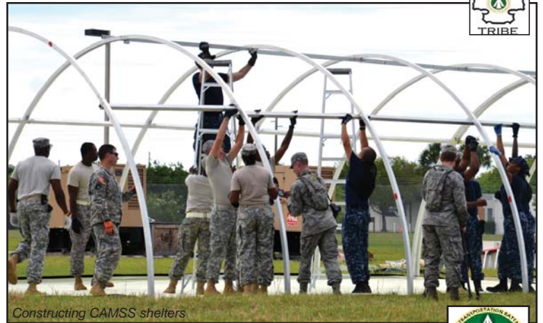
Constructing CAMSS shelters
