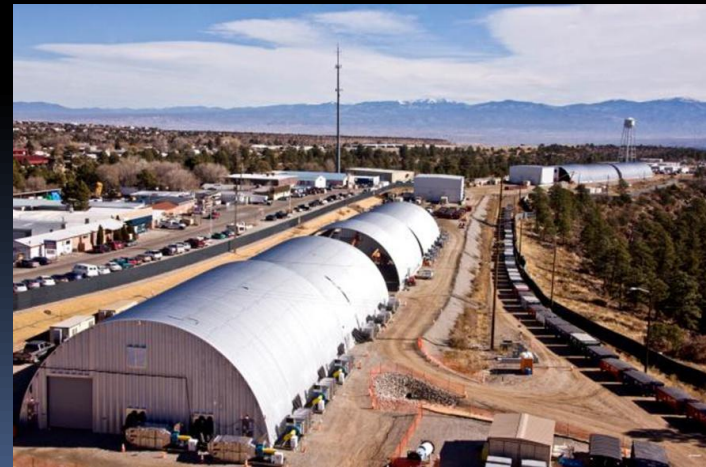
MDA-B Evacuation Area
