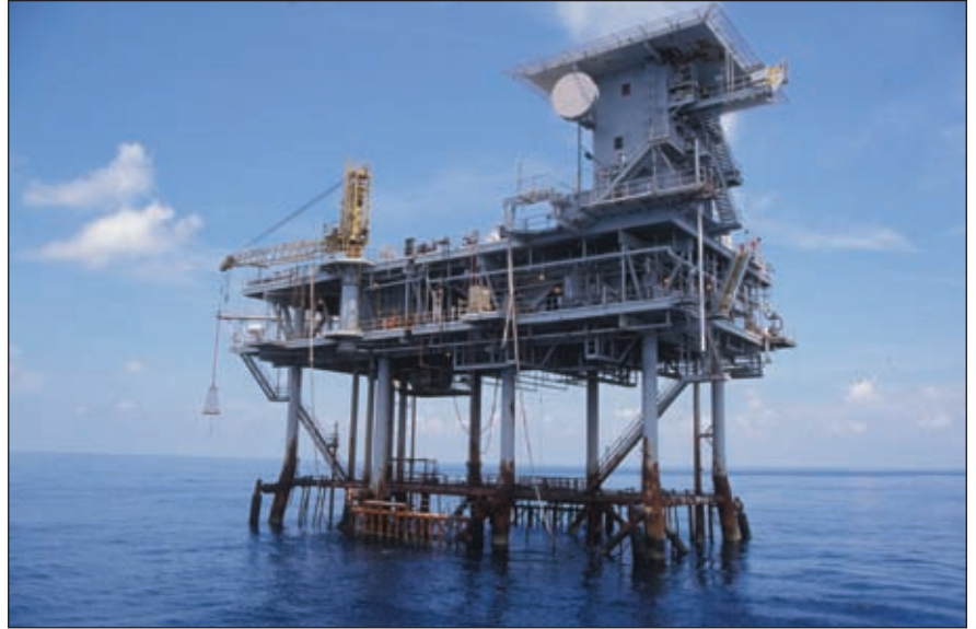
Figure 7.14. An operational gas platform within the boundaries of the FGBNMS. Photo: FGBNMS/G.P. Schmahl.
