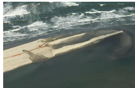
E4 North Berm Construction – August 31, 2010
