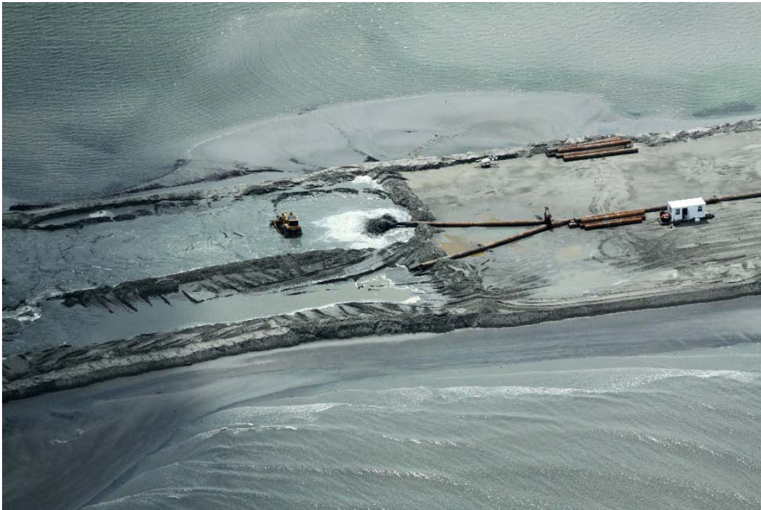
E4 North Berm Operations – August 18, 2010
