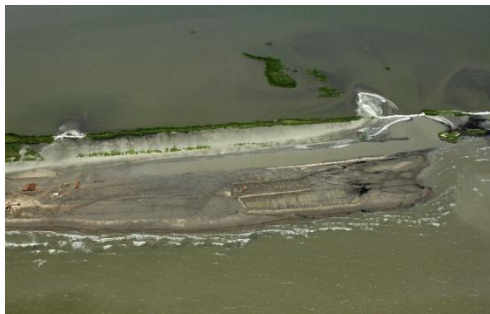
W9 Berm – August 18, 2010
