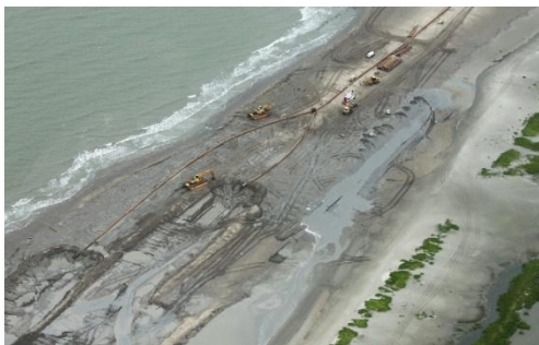
W9 Berm – August 15, 2010
