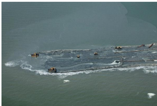
E4 Berm Construction – August 10, 2010
