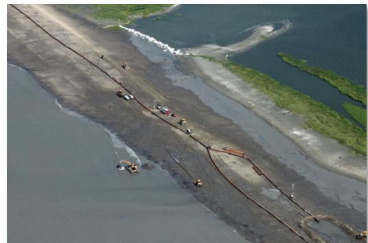
W9 Berm – August 10, 2010
