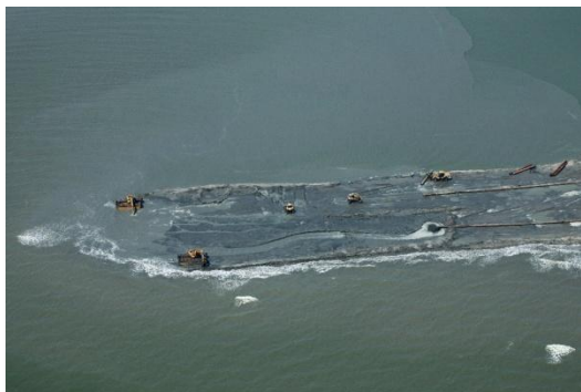
E4 Berm Construction – August 10, 2010
