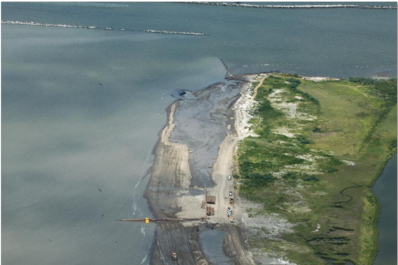
W9 Berm – August 1, 2010
