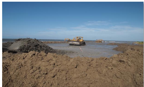
W9 Berm Construction – July 27, 2010
