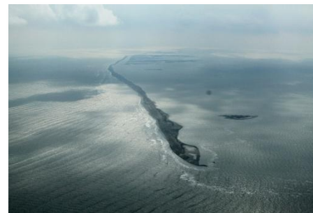
E4 North Berm – November 16, 2010
