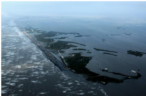
W10 Berm – November 16, 2010
